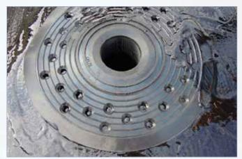
A second coat / layer of liquid membrane, or a patch of membrane in the case of torch-on-felt is installed on top of the flange to create an "over-and-under" bond so the outlet is bonded securely within the waterproofing membrane.
