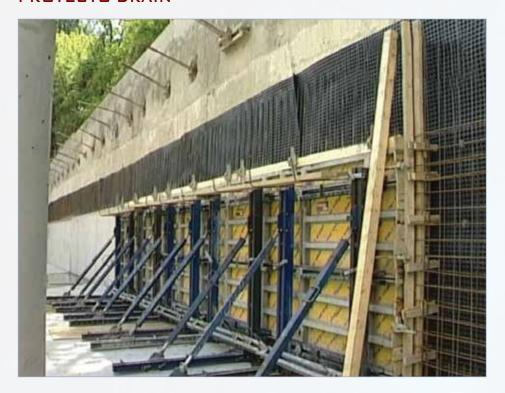
Protecto-drain is a preformed high density polyethylene (HDPE) membrane designed to protect surfaces and act as a drainage layer. It is manufactured with a series of cups and ridges to help channel water effectively.
