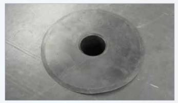
Waterproof the area around the drainage hole. Insert the correct size of outlet connector into the hole so that it is covering the waterproof membrane. Secure the connector either by using fixings or adhesive.
