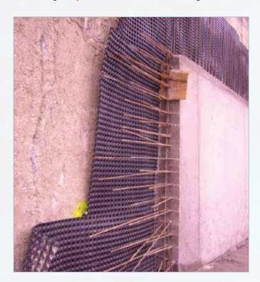
It is ideal as a lining membrane, as a waterproofing and protection layer between layers of concrete, on foundations, bridges and tunnels, and a whole manner of civil engineering works.
