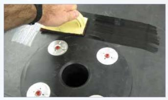
Prime the area and install another layer of waterproofing membrane, laid across the face of the outlet connector so that it is encapsulated in a "sandwich".
