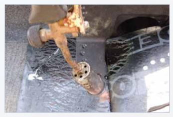
A second layer of felt is installed immediately on top of the flange (and the patch beneath it) whilst the bitumen is still tacky and is torch-heated so that the bitumen on this upper layer melts slightly. The two layers of felt adhere to each other, encapsulating the outlet.
