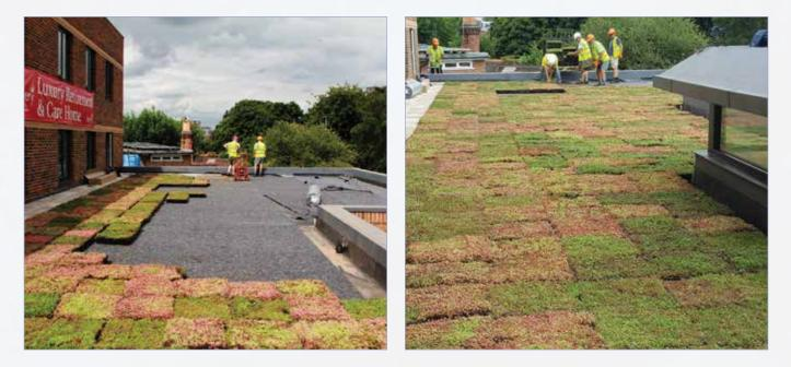
3. The edges should be filled with a border of washed riverstones, in accordance with the GRO code of practice. Objects such as roof lights and cables should be surrounded with riverstones to prevent root invasion and act as a fire break.
