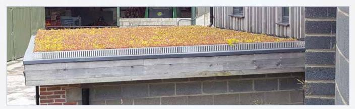
The profile is right angled, so it can sit underneath either the M-Tray® or the pebbles and be weighted down sufficiently.
