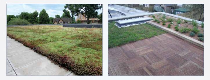
Areas such as paving or timber decking (laid onto Wallbarn ASP or TD pedestals) can be built up to the same height as the vegetation, creating one seamless garden level.
