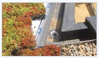
It can be mechanically fixed to the surface beneath, but if this is not possible due to the waterproofing membrane's integrity, the angle can be ballasted.
