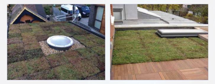
The modular sections mean detailing around objects is a simple process and clean lines are created. Hard landscaping sections such as paving and decking, mounted onto Wallbarn pedestals, can be added to the area to allow for regular access. As everything is suspended on top of the deck, drainage is uninterrupted.
