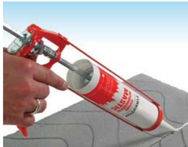
ROCKWOOL Acoustic Intumescent Sealant in blockwork joints
