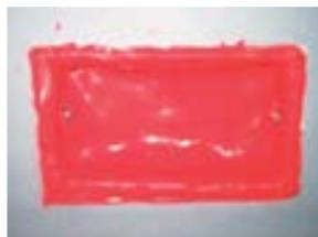
Putty Pad installed inside switch box
