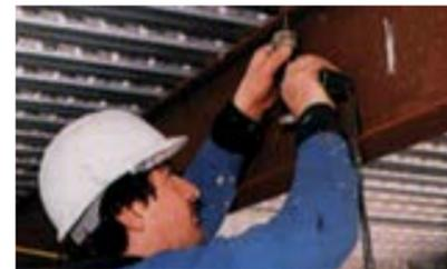
Fixing stud welded pins
