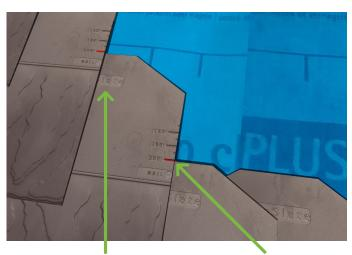
Each slate has embossed guidelines to aid location; the **vertical lines** at the top of the slate assist in locating slates horizontally. Horizontal lines on the edges are a guide for the overlap required dependant on pitch.
