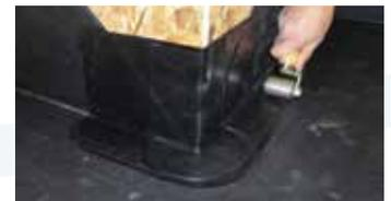
4) The finished corner will have 2 sections of tape of equal size overlapping each other by 75mm past the corner. Roll the entire corner to achieve full detail strength.
