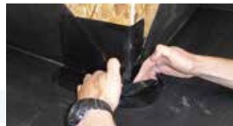
3) Once dry remove clear poly backing and adhere tape into position starting from the top of the tape and working down. Roll the tape then repeat the process from the opposite direction.
