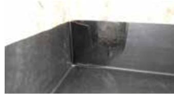
3) Apply ClassicBond Primer to the marked area (inside, outside of the flap & upstand) and allow primer to dry.
