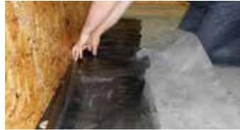
3) Test the Bonding Adhesive to ensure it has become touch dry. Next, work the membrane into the right angle and up the upstand.
