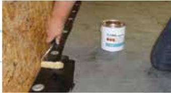
1) Apply ClassicBond Bonding Adhesive to the EPDM membrane and onto the exposed edge of the RUSS strip.
