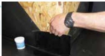
1) The membrane should be cut from the base of the corner to the top at a 45° angle. Use a section of PS Elastoform flashing to give 75mm coverage round the corner, 50mm past the top of the cut and up to 75mm onto the flat area. Put the tape in position and mark around it.
