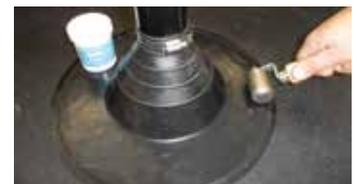
4) Remove the clear poly backing layer and mate the pipe seal onto the membrane. Roll the flat area of the seal to achieve full strength.
