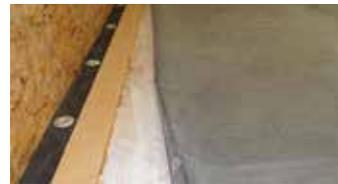
3) Lay the membrane into the ClassicBond Deck Adhesive when the adhesive is still wet. If using ClassicBond Bonding Adhesive allow the adhesive to become touch dry before mating the surfaces together.
