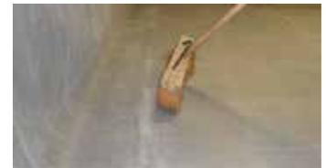
4) Push the EPDM membrane into the adhesive with a soft broom to remove any trapped air and achieve a complete bond. The membrane should be free of any wrinkles or creases.
