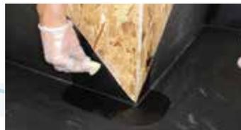
2) Apply ClassicBond EPDM Primer to the marked area. Primer should only be applied to dry and clean surfaces. You can apply ClassicBond Primer to a range of surfaces such as brick, plastic, timber etc.
