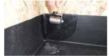
4) Once dry, remove clear poly backing and adhere tape into position. Roll the internal corner detail with a hand roller to achieve full detail strength.
