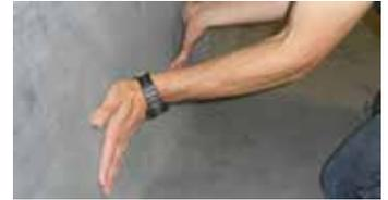
4) Mate the two surfaces together ensuring there is no trapped air under the membrane. If the membrane and substrate are put together when wet, bubbling will occur.
