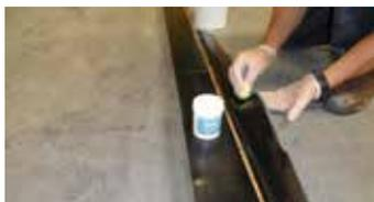
1) Adhere both sheets fully in position allowing the sheets to overlap by a minimum of 75mm. Apply ClassicBond Primer to both the bottom overlap area and to the underside of the top lap.
