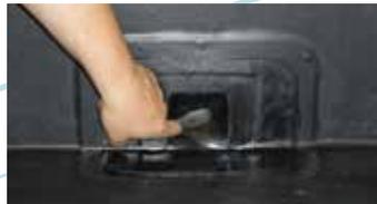
2) Install a section of 225mm PS Elastoform tape to the primed area. Cut a small hole in the tape and form it into the opening.
