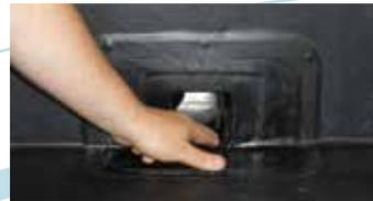
3) Prime inside the outlet for installing a securing strip of tape. Install a strip of PS Elastoform flashing 75mm wide around the inside of the outlet opening to secure the flashing in place.
