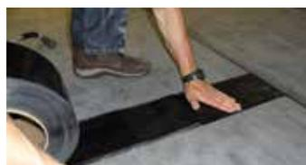
3) Once the primer has become dry, unpeel a section of the clear poly backing and start adhering the tape to the primed area with a flat hand. Ensure there is no trapped air in the seam.
