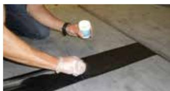
2) Prime a strip 80-90mm either side of the joint with ClassicBond EPDM Primer and allow the primer to become touch dry.
