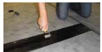
4) Roll the entire seam with a hand roller, rolling at right angles to the seam not along it, to achieve full seam strength. 225mm PS cover patches must be applied at seam junctions.
