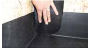
2) Cut a section of 225mm PS Elastoform flashing to give 75mm coverage past the edge of flap and large enough to extend up to the top of the corner. Put the tape in position and mark around it.
