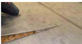
1) When installing a 150mm Cover Strip as a butt joint, adhere both sheets in the required position. Ensure there is no gap between the sheets.
