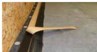
2) Once the ClassicBond Primer has cured, remove the protective strip from the PS tape section of the RUSS strip.
