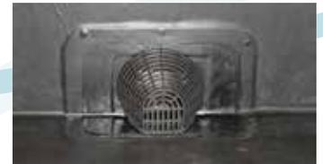
4) Roll the entire flashing with the hand roller and install leaf grate.
