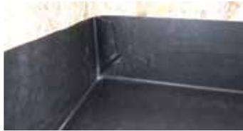
1) Adhere the membrane to the upstands (see section C) and fold the membrane together to form a triangular flap. Fold the flap back to one side and trim any excess membrane away leaving a flap approx. 75mm wide.
