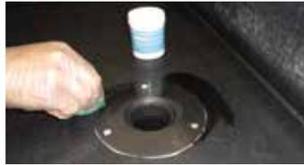
2) Apply ClassicBond Primer to the head of the outlet, down into the outlet pipe and onto the membrane around the outlet.
