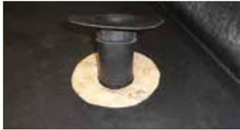
1) Cut the head of the outlet back to leave a 50mm flange around the outlet hole and fix into the decking. Cut the membrane around the perimeter of the outlet head.
