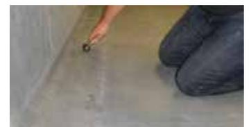
4) Using a hand roller, roll the membrane into the PS RUSS strip to achieve the full bond.
