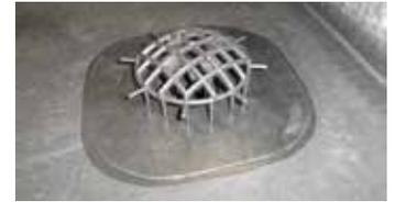
4) Cut an opening in the centre of the tape and form the tape into the outlet by 15mm. Ensure the entire flashing has been rolled and install the leaf grate.
