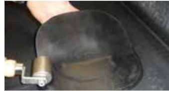
3) Allow the primer to dry and adhere a section of 225mm PS Elastoform tape to cover the outlet and seal onto the ClassicBond EPDM membrane by at least 50mm.
