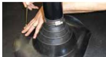
2) Fit the metal clamping ring to the pipe boot. Mark the ClassicBond EPDM membrane around the base of the pipe seal to give a guide for applying the ClassicBond Primer.
