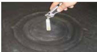
1) Fix the outlet into the deck and put the protective yellow cap into position. Install the membrane over the top of the outlet. Find the locating pin on the outlet cap, place the cutting guide over the pin and cut away the circle of ClassicBond membrane.
