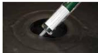
3) Put a bead of ClassicBond water cut off mastic inbetween the EPDM membrane and the top of the outlet.
