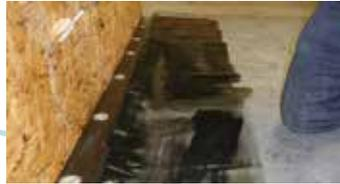
2) Bonding Adhesive must also be applied to the vertical surface. This must be clean, dry and free of any sharp protrusions. Allow the Bonding Adhesive to become touch dry.
