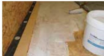
2) Apply ClassicBond WBA Deck Adhesive to the roof deck up to the edge of the RUSS strip. If installing with ClassicBond Bonding Adhesive, apply to the substrate and to the underside of the membrane.
