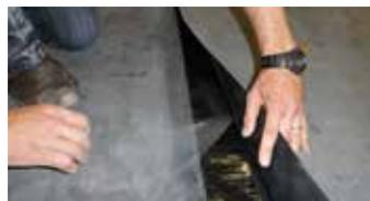
3) Once the 75mm tape is bonded to the bottom sheet, fold over the top lap to cover the seam and remove the clear poly backing protective strip and smooth the primed top lap onto the tape.
