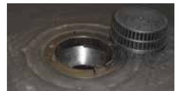
4) Securely screw in the clamping ring. Once the clamping ring is fully tightened, clip the leaf grate into its three locating tabs.
