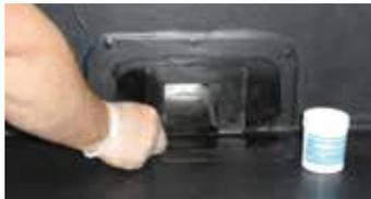
1) Install the membrane over the top of the outlet and cut the membrane 25-50mm around the outlet hole. Prime the outlet and the membrane around the outlet with ClassicBond EPDM Primer and allow to dry.
