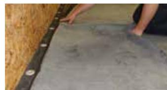
3) Lay the primed area of the ClassicBond EPDM membrane onto the exposed PS tape on the RUSS strip.
