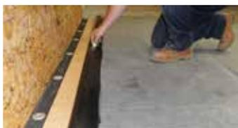
1) Fold the membrane back and apply ClassicBond EPDM Primer to the area of EPDM membrane that will mate into the 75mm wide PS tape on the RUSS strip and allow to dry.
