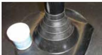
1) Using a pre-formed ClassicBond PS pipe seal, cut the seal at the top to the correct size for the pipe. Always cut above the rib on the pipe seal.
