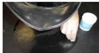
3) Apply ClassicBond EPDM primer to the membrane in the marked area and allow to dry become touch dry.
