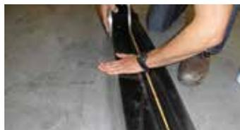
2) Once the primer has become dry, unroll a section of tape and position it onto the primed area of the bottom sheet. Continue adhering the tape along the entire seam ensuring there is no trapped air.
