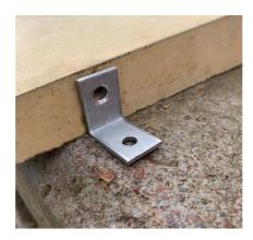
Drill the holes as required using an 8mm masonry drill and fit the Duopower plugs. The brackets can now be screwed into position with the stainless steel screws provided. When installing the pins we recommend resin bonding the pins into the holes.
