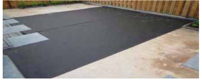
Step 2 – Apply Membrane/Pressure Distribution Cloth
