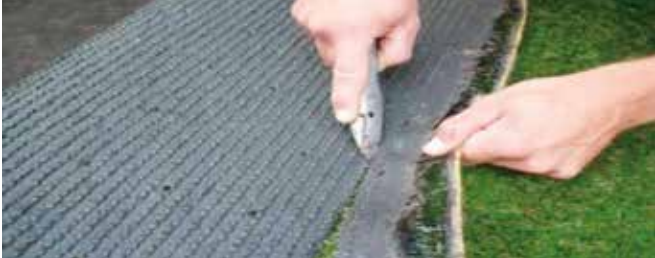
Step 3 – Cut Artificial Grass To Size
