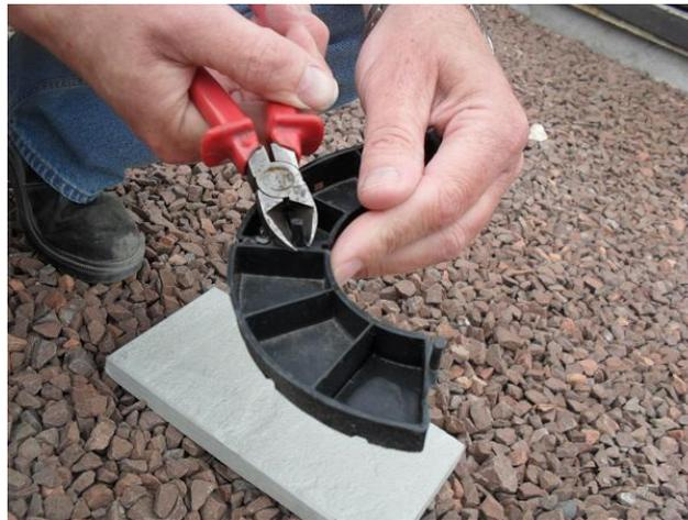
If there are any obvious high points on the roof then it may be necessary to start from that area so that the lower areas can be lifted by levelling discs. If necessary the PSP's can be stacked up to four high to overcome undulations in the roof surface. PSP's are available in 12mm and 15mm and the levelling discs are available in 1, 2 and 3mm.
