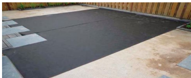
Step 2 – Apply Membrane/Pressure Distribution Cloth
