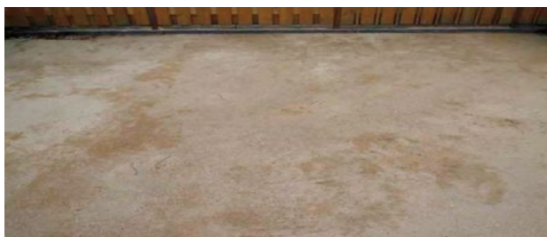
Step 1 – Apply Foundation For Artificial Grass
