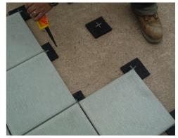
Cutting is easily achieved using a diamond blade on a cutter/grinder. When cutting tiles ensure that dust created is not allowed to build up on completed areas as staining may occur.
