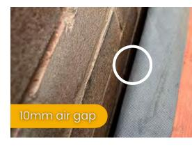
**4** Double Batten the Area: Install double battens at least 10mm away from the wall to provide additional support for the sheets.
