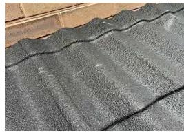
5 Install the Pantile 2000 Sheets: Place the Pantile 2000 sheets on the roof area, ensuring they are positioned up to 10mm from the wall. Secure the sheets with main fixings into the timber purlins below.
