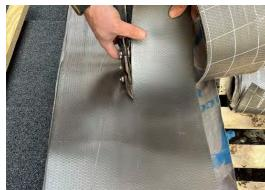
6 Install the LEADAX Flashing: Insert the LEADAX into the scribed area, ensuring it is dressed down flush against the wall and extends over the upstand of the sidewall flashing.
