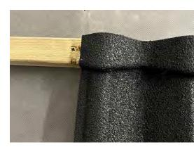
2 Position the First Sheet: Lay the first sheet from right to left, ensuring it reaches up to the batten.
