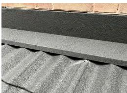
**8** Seal the Scribed Area: Apply silicone sealant to the scribed area, matching the colour of the flashing for a finished look.
