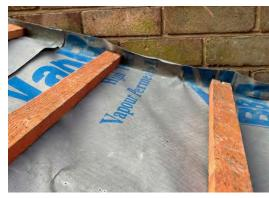
2 Measure and Scribe: Measure and mark a line 150mm above the battens, extending the full length of the rafter. Scribe along this line to a width of 2-3mm and a depth of 25mm.
