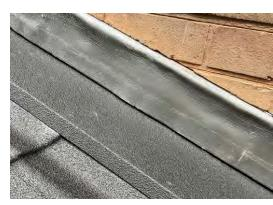
7 Seal the Scribed Area: Apply silicone sealant in a matching colour to the scribed area to ensure a watertight seal.
