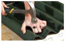
Plastic capped Monobloc nails Fix by striking the preformed Monobloc head with the hammer through the top of the corrugation. Note: You do not have to pre-drill the sheet.
