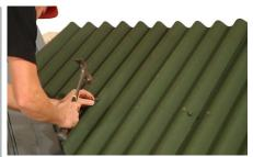
**Fixing sheet to valley**The fixings to the roof sheets can then be applied.
