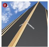
Build up the ridge batten using 25mm thick battens to the required height, usually two battens are sufficient for most profile tiles. Secure the battens in place using the stainless steel batten straps provided. Where Easy-Verge U is to be installed, the ridge batten must extend beyond the ridge by 30mm at each gable end.
