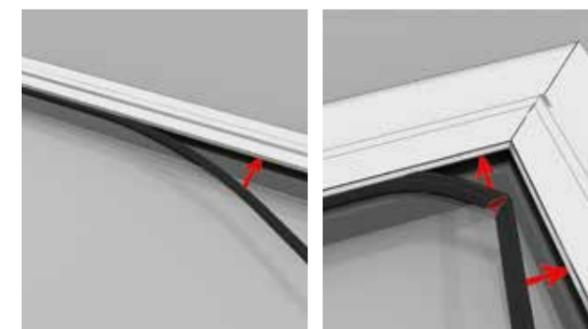
**8** Starting from a corner, apply the wedge gasket to the opposite side of the vent sash (to the glazing tape), notching the corners to allow the gasket to fit tight into the corners of the framework.
