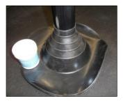
1) Cut the <u>ClassicBond PS Pipe Seal</u> above the raised "rib" one size smaller than the pipe diameter. DO NOT CUT THROUGH THE RIB. Pull pipe seal over pipe until base flange is in contact with the ClassicBond EPDM membrane.
