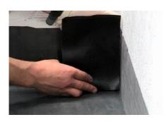
2) Cut an appropriate size piece of 225mm uncured flashing (min. 50mm wider than the flap of membrane), press the flap back to the upstand and install the uncured flashing tape.
