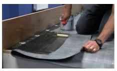
4) Once bonded to the RUSS finish the upstand by using Bonding Adhesive to the remainder of the RUSS, upstand and membrane.
