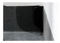
1) The fold should be cut back to leave a 75mm wide flap. Apply ClassicBond EPDM Primer to the front & back of the flap and to the membrane on the wall. ClassicBond Primer must be allowed to dry before application of PS tape.
