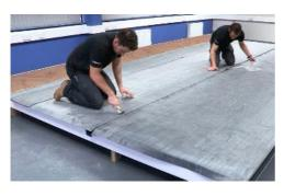
3) Lay the top membrane onto the Seam Tape. Pull away the poly backing from the tape at a 45° degree angle to the seam. While removing the poly backing, draw your hand across the seam, from the back to the leading edge. Roll the seam at right angles to the seam direction, not along it.
