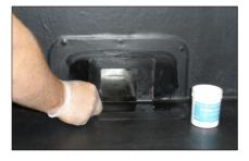
1) Install outlet into parapet wall before installing EPDM membrane. Install the ClassicBond EPDM membrane over the outlet with ClassicBond Bonding Adhesive. Cut the EPDM membrane away from outlet opening by 50mm. Apply ClassicBond Primer to the membrane, outlet face and into the outlet pipe.
