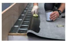
2) Apply ClassicBond Primer to the area on the underside of the EPDM membrane that will come into contact with the 75mm PS tape on the RUSS strip.
