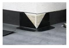
2) Apply ClassicBond Primer to the marked area to be flashed and allow to dry. The area must be clean and dry before application of primer, apply primer to membrane and to upstand substrate. ClassicBond Primer must be allowed to dry before application of tapes.
