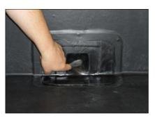
2) Install Uncured PS tape to the outlet. This should be large enough to join onto the membrane by a minimum of 50mm. Cut a small square out of the middle of the tape and mould the tape into the outlet pipe by 25mm. Cut a second section of Uncured PS tape 100mm wide. This will be inserted into the outlet pipe to reinforce and lengthen the tape that was turned into the pipe by 25mm. Apply
