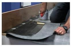
1) Apply the Bonding adhesive to the side of the RUSS strip or exposed decking. Also apply the Bonding adhesive to the relevant upstand termination or step down and to the back side of the ClassicBond membrane
