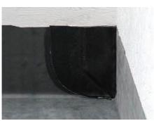
3) Roll the taped area with hand roller once installed.
