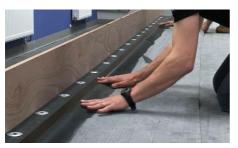
3) Once the primer is dry remove the protective strip from the PS tape on the RUSS strip. Lay the primed membrane into the PS tape with no wrinkles or air gaps and smooth in by hand then roll with hand roller.
