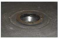
3) Insert a bead of <u>ClassicBond Water Cut</u> <u>Off mastic</u> between the underside of the membrane and the top flange on the outlet. Screw in the clamping ring till it's completely tightened. Use the two tightening lugs to apply leverage to the ring.
