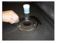
1) Cut the outlet flange back to leave a min. 50mm head and cut the membrane back to meet the perimeter of the outlet head. Secure the outlet into the decking and apply ClassicBond Primer to the head of the outlet and to the EPDM membrane.
