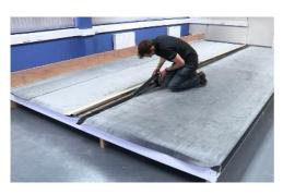
2) Using moderate pressure set the Seam Tape into place to keep air from being trapped under the tape and unroll the 75mm wide tape along the length of the seam, aligning the Seam Tape (not the clear backing) along the chalk line. Care must be taken not to get any bubbles or wrinkles in the tape.
