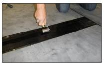
4) Once the entire length of tape is applied to the seam, roll across the 150mm tape with hand roller. Where 150mm tapes intersect other tapes, 225mm uncured tape cover patches must be applied.
