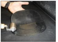
2) Apply the Uncured PS tape to the primed area. Once fitted cut a small section from the centre of the tape out to expose the outlet opening and press the remainding tape down into the outlet. Roll the entire flashing with hand roller.
