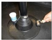
3) Pull pipe seal back down over pipe and into position. Remove poly backing from the tape and with hand pressure press tape onto primed area. Roll splice area with a hand roller
