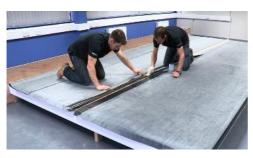
1) Fold the top sheet back to expose the seam area. Using a scrubbing pad apply the ClassicBond Primer to the seam area. Apply the primer past the seam edge to the line. ClassicBond Primer must be dry before application of PS tapes. NOTE: If the EPDM membrane is contaminated with dirt, etc., clean the seam area.
