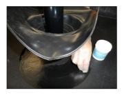
2) Once in position clamp the seal to the pipe with the supplied metal clamp and mark around the base of the seal to give a line to prime up to. Pull pipe seal upwards on pipe to expose the membrane and apply ClassicBond EPDM Primer to the EPDM deck membrane
